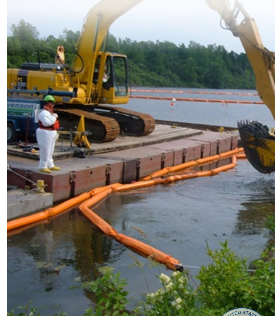
Photo Source: Anchor QEA
