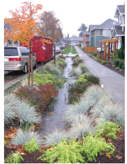
Bioswales retain and treat stormwater in High Point
